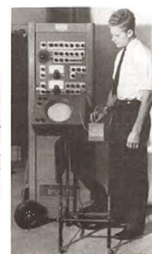
Fig. 21. Type A supersonic reflectoscope.
