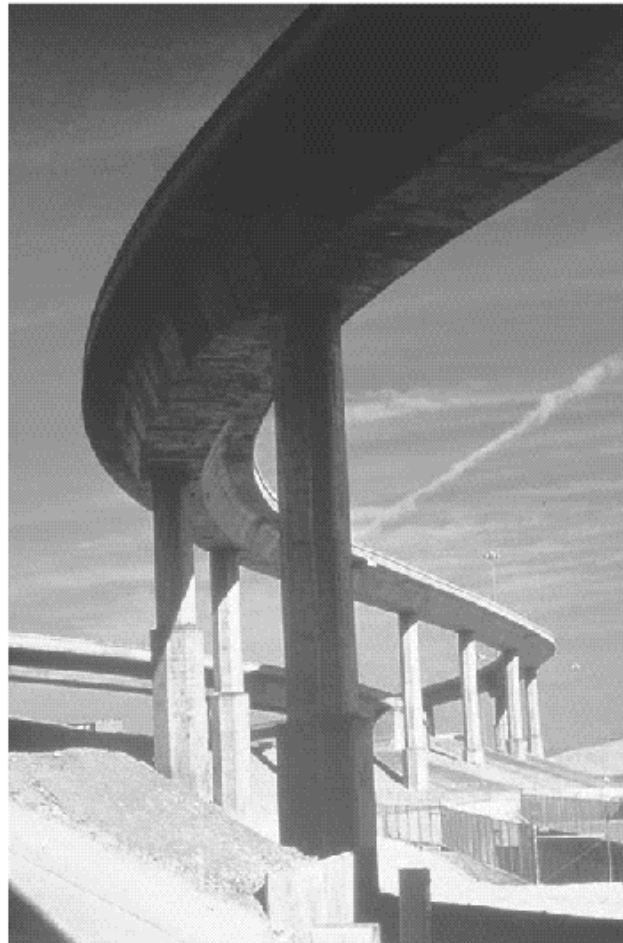
FIGURE 7.2 Curved continuous beam bridge, Las Vegas, Nevada, designed for torsional effects. (Courtesy of Portland Cement Association.)
