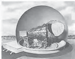
FIGURE P5.9 A model of the antenna for the Telstar System at Andover, Maine. (Photo courtesy of Bell Telephone Laboratories, Inc.)
