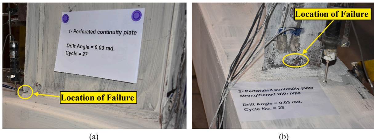
Fig. 29. Location of failure on the beam flange: a) Specimen 1(ID); b) Specimen 2 (SID).
