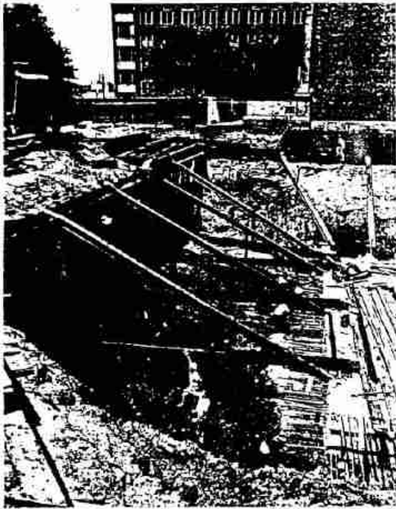
Fig. 13.25 Excavation for M.I.T. Center for Advanced Engineering Study.
