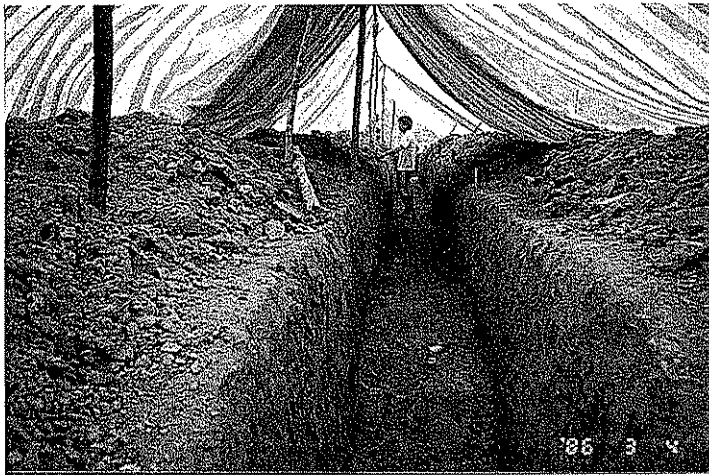
Figure 4.17. Inspection trench across the test field with shelter (courtesy of LI).
