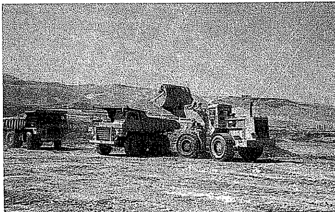
Figure 9.2. Earth moving work using wheel loader and dump trucks.
