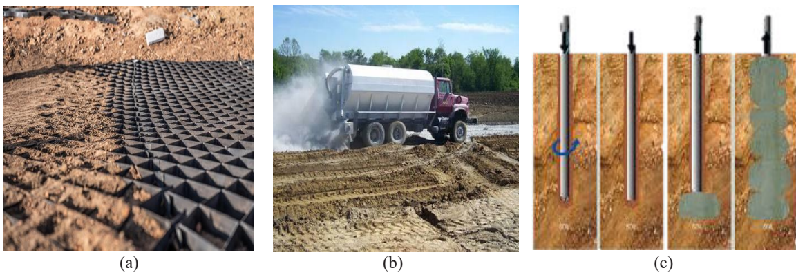
Figure 1-1. Some of the soil stabilization methods, (a) Geocell, (b) surface chemical stabilization, (c) deep mixing method
