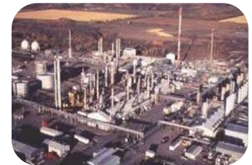
natural gas processing
