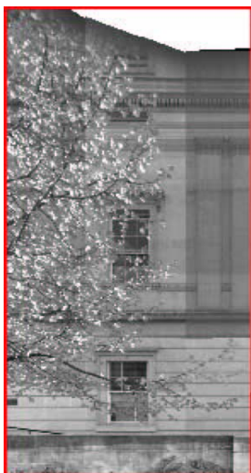
Figure 5. Texture with a missing part.
