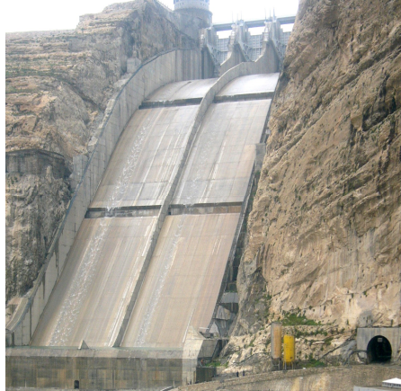
Figure 1: Spillover of Marun dam
